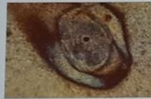
Pinhole corrosion - Chloride ions
